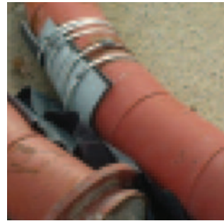
Example of a pipe that has perforations on the steel casing showing an attachment of a temporary patch preventing material escaping to atmosphere
